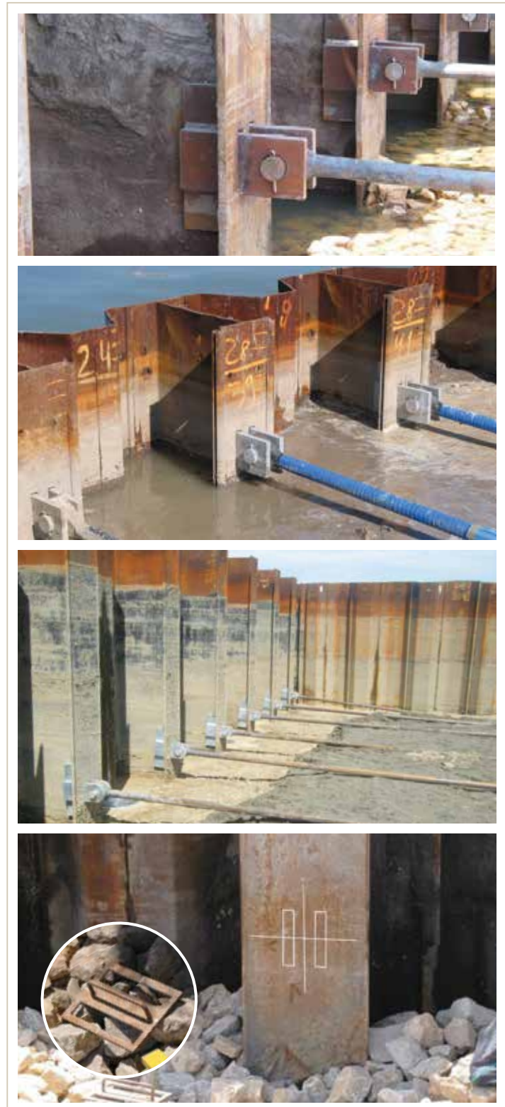
Fig. 5. Installation of the T-connectors at the job-site.
