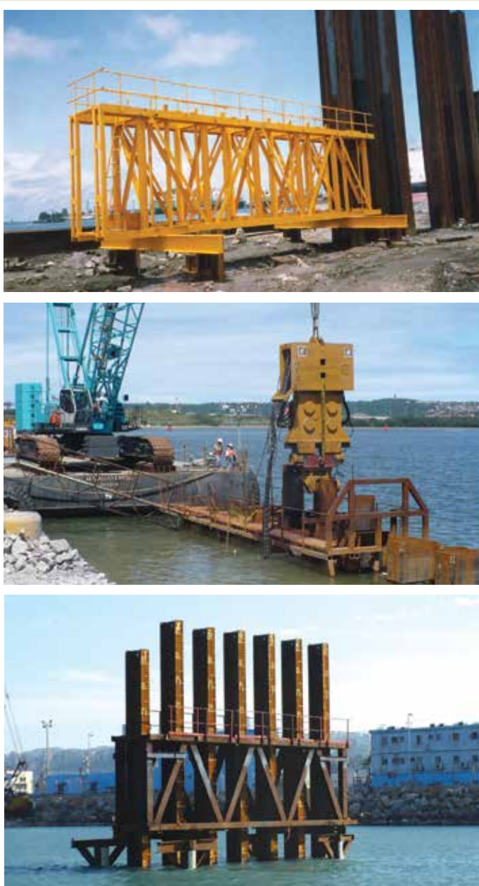
Fig. 9. Driving templates and their support.
