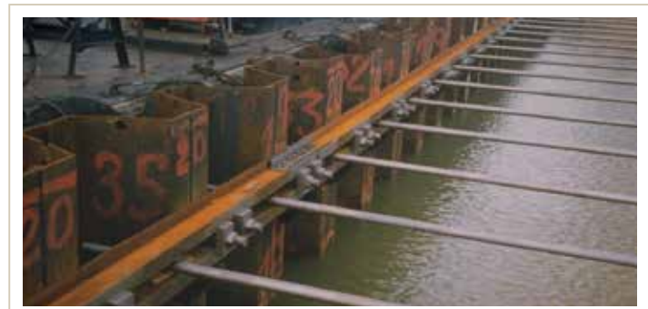
Fig. 6. Conventional anchor solution with tie-rods, walers, ...
